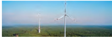
WIND-HYDRO HYBRID: GAILDORF, GERMANY The first wind farm with an integrated hydropower plant.
