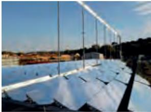
SUNCNIM CSP demonstrator operating automatically at the Seyne-sur-Mer since 2010
