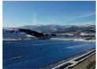
eLlo: CSP plant in the Eastern Pyrenees, France, 9MWe with 4 hours thermal storage (under construction)
