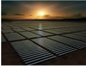
PRIESKA, SOUTH AFRICA: 75 MW
