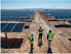
PV SALVADOR, CHILE: 68 MW
